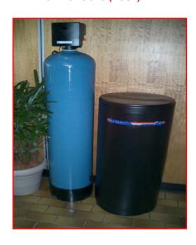
Fleck 5000SE electronic 5 stage regeneration fully adjustable functions Microprocessor control
